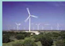
Courtesy of General Electric
